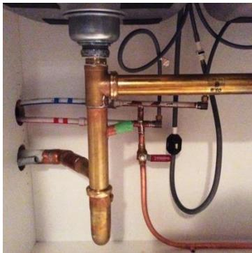
As noted in the Appliance section, the shut off valve for the dishwasher is also located below the sink on the copper line feeding the dishwasher.
